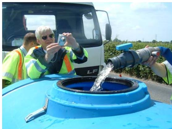
Figure 8b Clear water, 5mins after the ice pig
